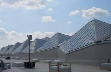
The solution chosen was to connect the upper translucent surface with the steelwork below using short tubular legs, so the two structures are close enough to give the desired effect. The solution used is a complete and tested "roof system". An exclusive system including aluminum profiles, with special joint and adjustable brackets, specifically designed by the company Lazzaro Srl.
