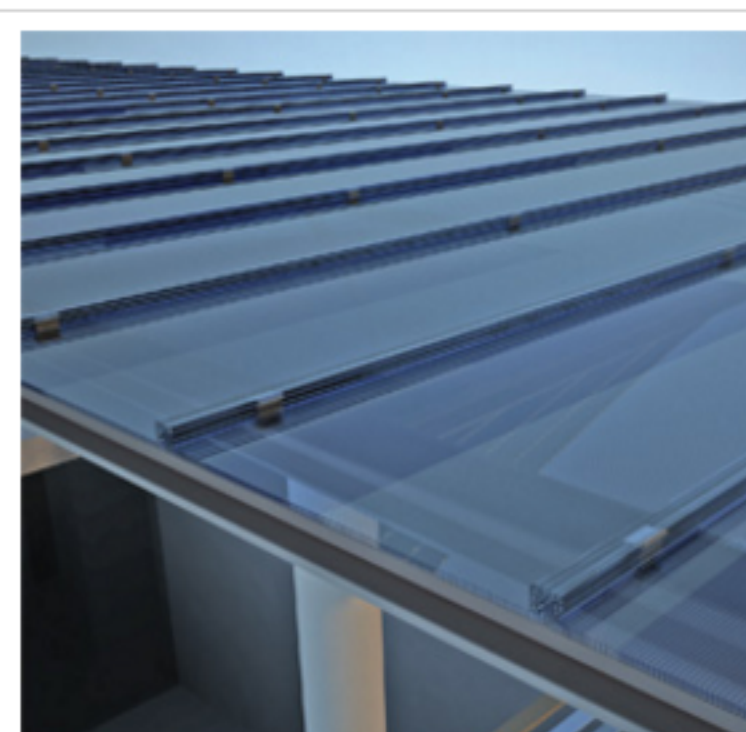
Example of roofing with polycarbonate cover plate
